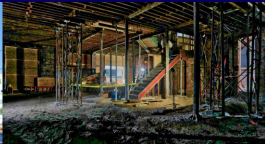
The entire concrete slab was demolished with no damage to the foundations or walls.
