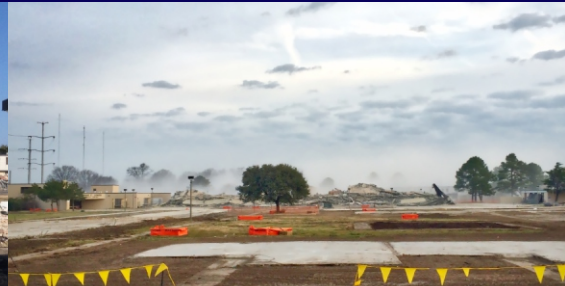
Eight story building entirely demolished by implosion in fifteen seconds.
