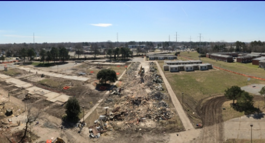
Eight story building entirely demolished by implosion in fifteen seconds.
