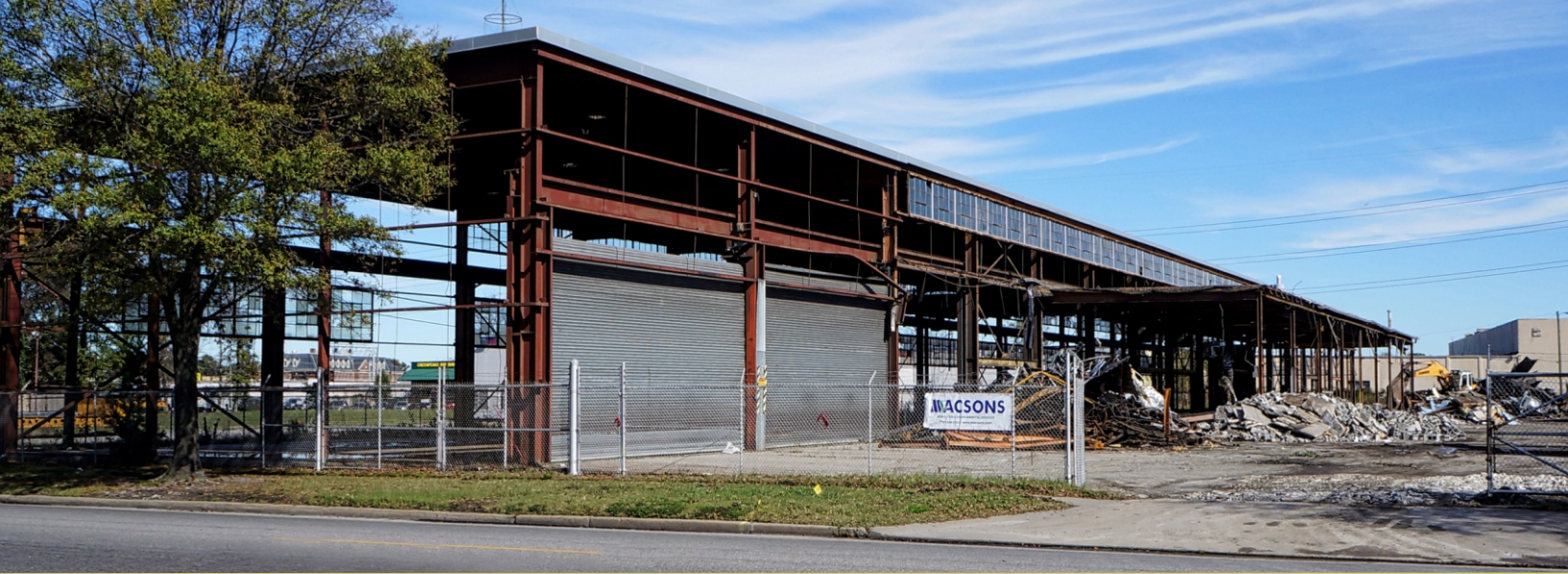
Exterior asbestos paneling (shown below left) was fully removed prior to demolition.
