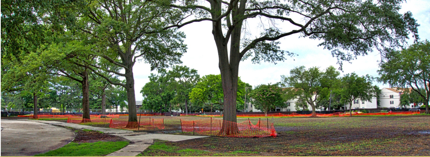
Clear Field: Abatement & Complete Removal; Ready for New Construction
